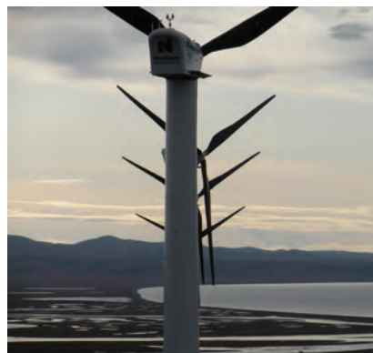
Six Northwind 100 turbines are providing power in Unalakleet.
