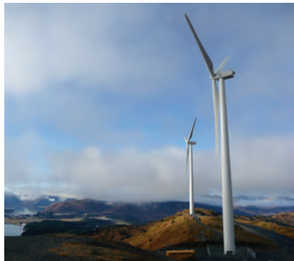
Three GE 1.5 MW turbines produce 9% of Kodiak's electricity.
