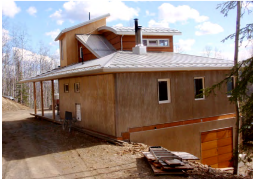
Figure 8. A view of the north side of the house. Note the near absence of windows on the north side (a good thing!) and the various roof lines (complicated!). The metal roof has snow “jacks,” also called snow stops, to prevent snow from sliding off the roof so that spring snow melt can be collected into a future cistern system for nonpotable uses.
