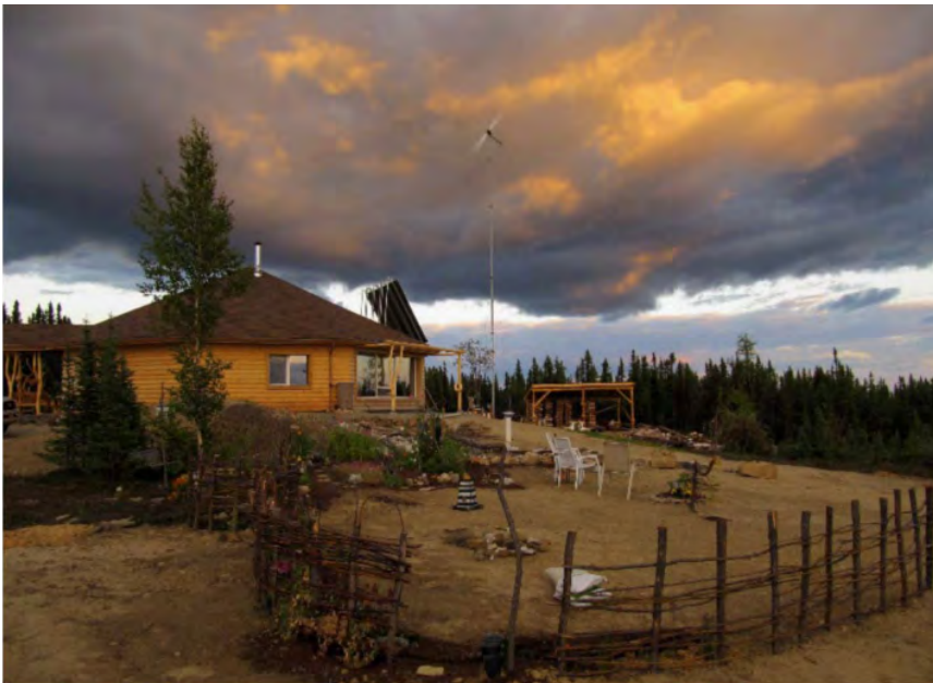
Figure 1. A view from the west of Karl Kassel's home. Note the large window area for passive solar gain. The siding is log siding (the house is not a log structure). The walls are insulated with Styrofoam insulation and are rated at R-65. There is no basement or crawl space. The house is built on the surface of the soil and insulated under the concrete floor with Styrofoam as well. Note, too, that the site is fairly windy, a fact I gleaned from the lack of snow on the roof when I visited in winter. Normally, one would expect to see major snow accumulation on the roof, but that is clearly not the case for this location, which is on a ridgetop northwest of Fairbanks.
