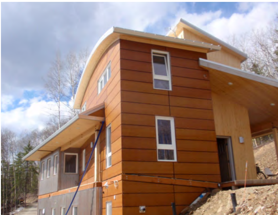
Figure 12. Another exterior view of the Reed/Wright home. The home has fiberglass windows all around and one of the tilt-turn windows is open for ventilation (third floor) in this photo. Note also the vent/exhaust on the east side of the basement floor, which is for a Toyotomi fuel-oil-fired heater used for back-up heat. This is ultimately to be displaced to the degree possible by the solar collection of heat. The site also has many years supply of wood for the masonry stove, so that minimal fossil fuel will be needed.
