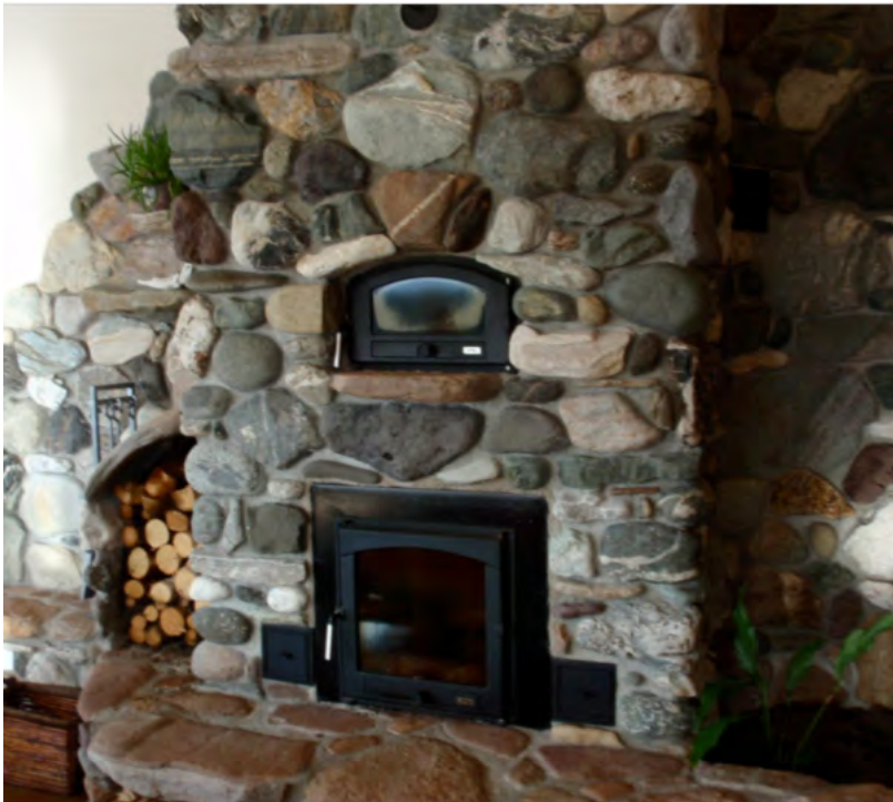
Figure 2. The masonry stove in Karl Kassel's home. The stones are all from the local region. The main firebox is the lower door, and the baking oven is the smaller upper door. The strategy of operation for this type of stove, which has firebrick and refractory (a high-temperature ceramic fire box lining) inside the firebox, is to burn fuel quickly at very high temperatures. As the stove heats up, flue gases pass through a series of serpentine channels inside the stove before exiting, transferring heat to the large mass of the stove (typically around 10-12,000 pounds of concrete and stone) and lowering the exhaust temperature to around 110°F. Heating the fuel, typically wood, to this high temperature allows full combustion and results in the very clean burn characteristic of masonry heaters.
