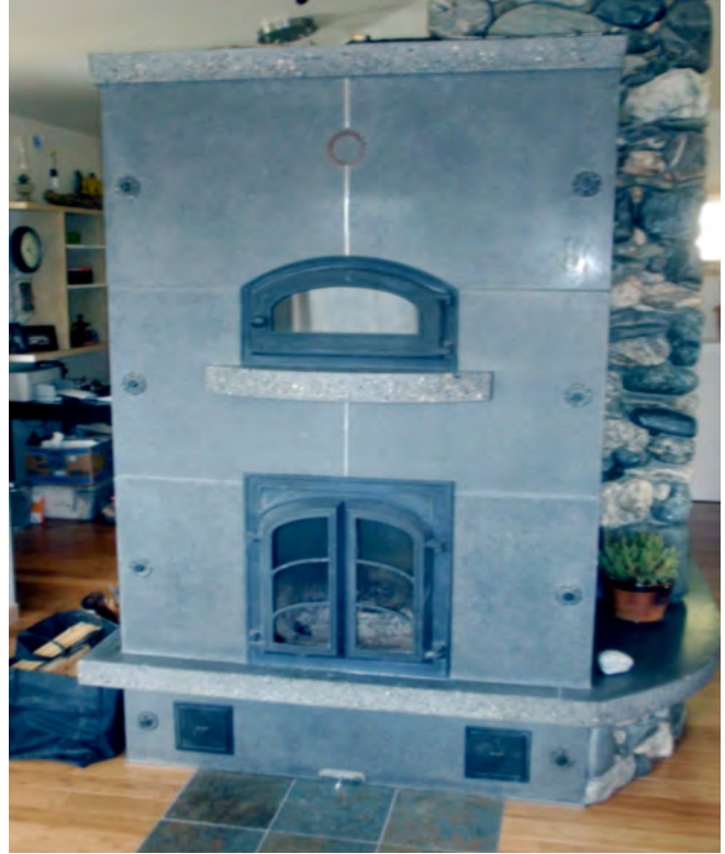
Figure 10. The front of the masonry heater in the Reed/Wright home.
