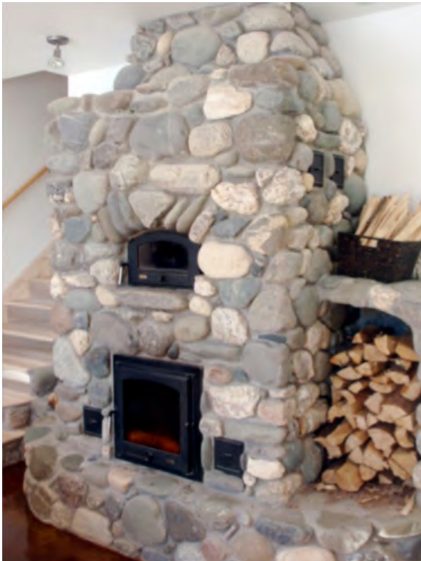
Figure 4. The masonry heater in the Chlupp home, also built by Dan Givens.
