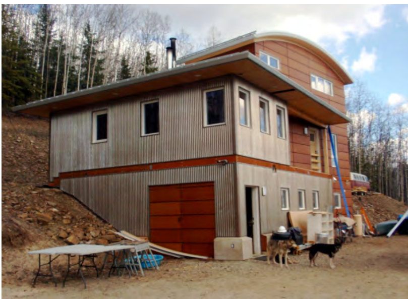
Figure 7. A view of the Reed/Wright house from the southwest. Two types of exterior siding are used. One is a corrugated metal siding with an oxidizing finish that “rusts” to form a protective, completely maintenance-free surface and is very weather-tight and durable. The other, a brown, woodlike siding, is actually a cementitious siding with a wood grain finish on it, and it is fire-proof and durable as well. These sidings were selected, along with yellow cedar decking, because of their ability to weather/age aesthetically while eliminating effort for reapplication of potentially toxic, costly, petroleum-based protective coatings. The house is three stories and will ultimately have solar flat-plate collectors for heating and hot water.
