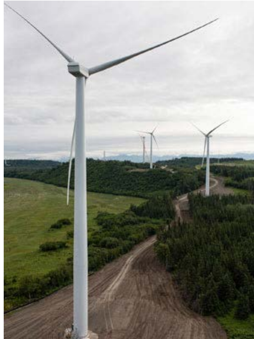
Fire Island Wind Project
