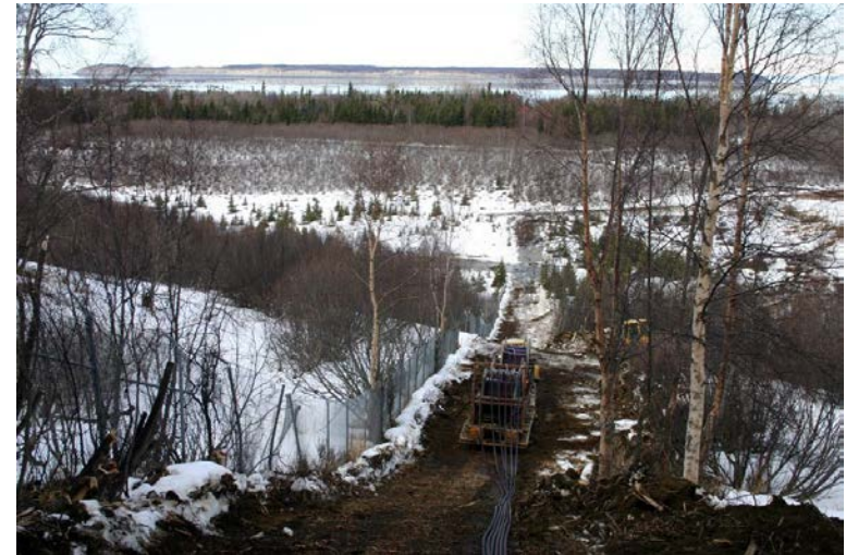
Cable bury at Point Campbell near Kincaid Park
