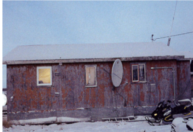
Quinhagak home before Weatherization program Energy Efficiency measures.
