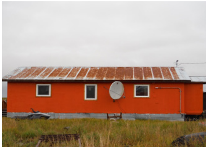
Quinhagak home after Weatherization Program Energy Efficiency measures.
