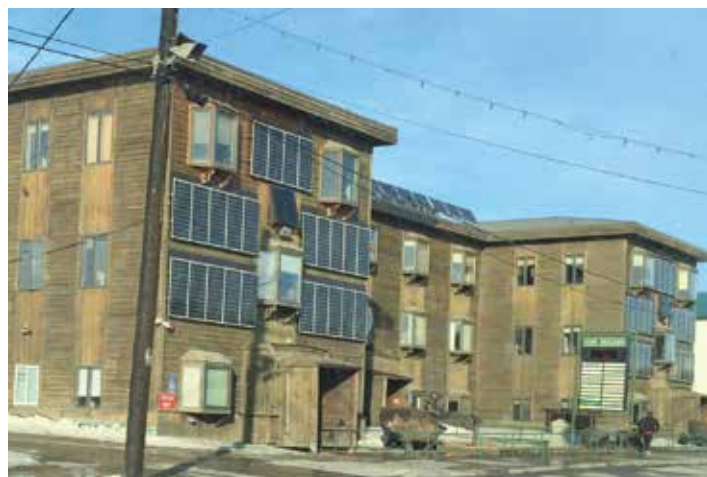
Solar panels are positioned to capture the low angle of the sun in Noatak (left) and Nome.
