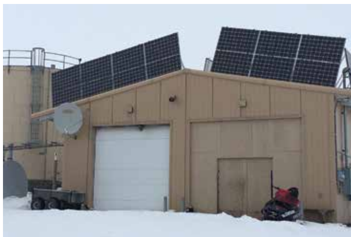
Solar panels are positioned to capture the low angle of the sun in Noatak (left) and Nome.
