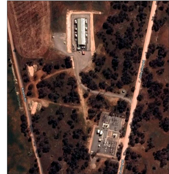
BESS and Dalrymple substation
