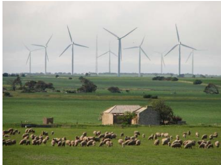
Wattle Point Wind Farm 91 MW (55 x Vestas V82 directly coupled induction generators)
