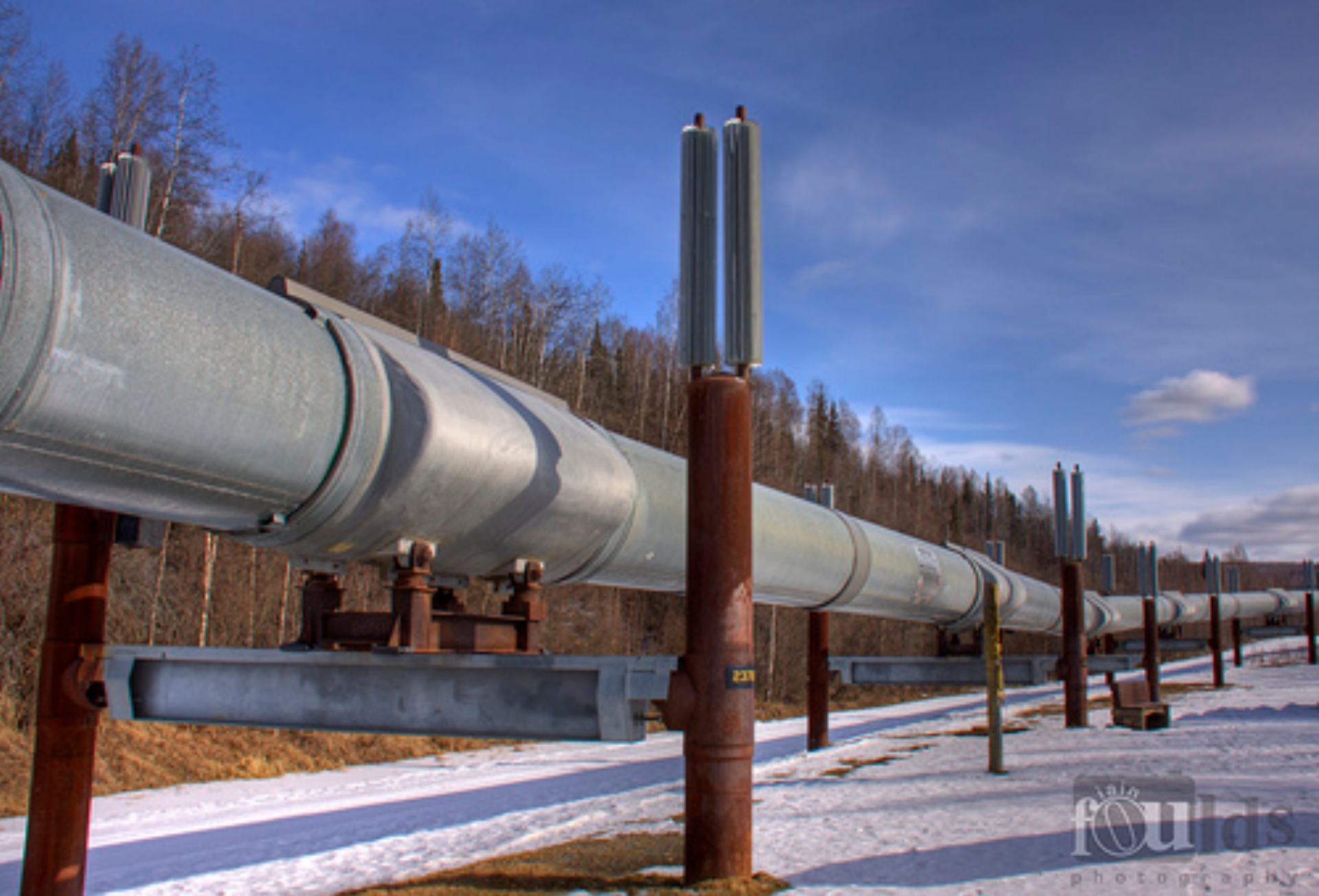
Trans Alaska Pipeline System
