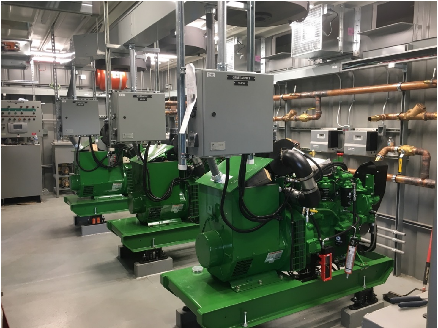
Port Heiden Power Plant Module Build and Imaging
