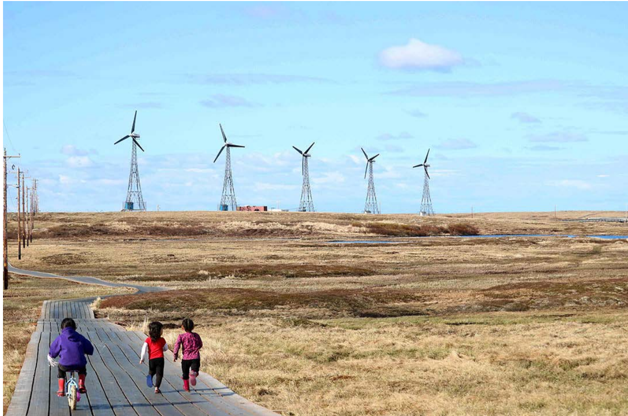
Figure 6. Kongiganak’s five Windmatic wind turbines, as seen from the town’s boardwalk. Image from Grainger (2022)
