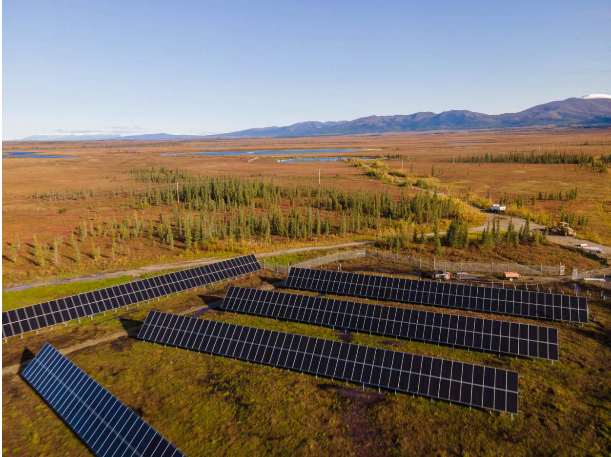
Figure 4. The 223.5-kW solar PV array that powers Shungnak and Kobuk. Image from DeMarban (2022)
