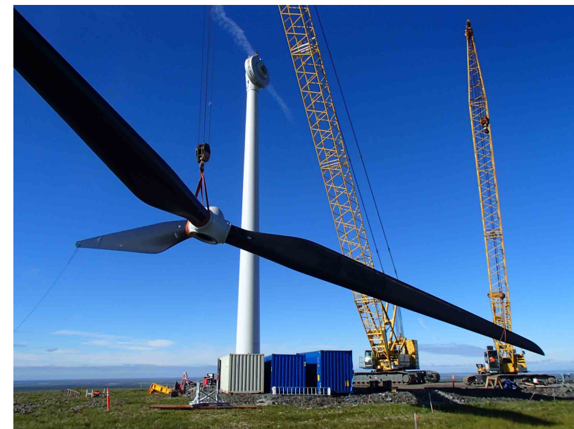
EWT 900 kW model DW54 900HH50 variable-pitch turbine
