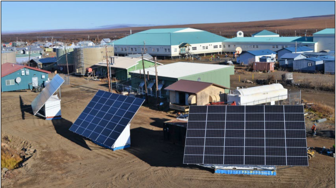
Figure 28. Buckland Solar Array
