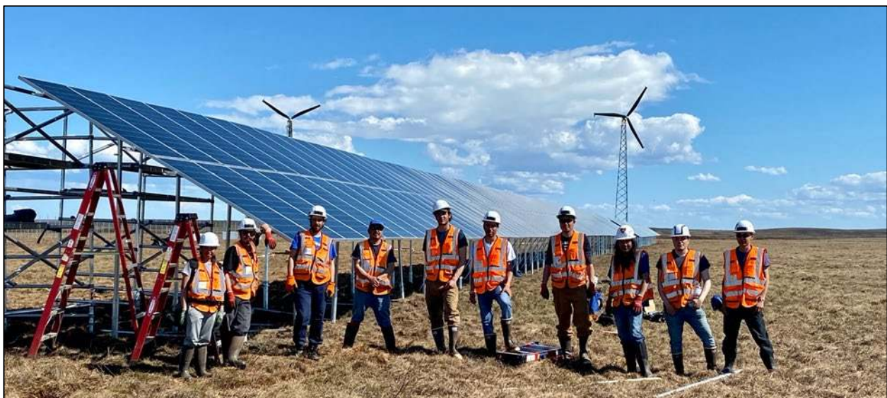
Figure 2. Solar Installation Crew in Kotzebue (Photo Courtesy of Matt Bergan)
