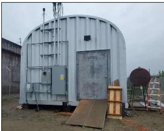
Figure 29. Shungnak Battery Building (Photo Courtesy of Ingemar Mathiasson)
