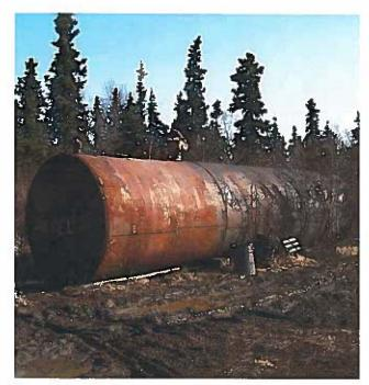
Typical non-code compliant bulk fuel tank that requires replacement.
