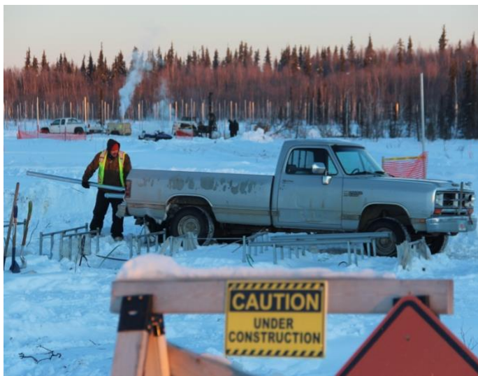
Construction underway on a solar project in Galena, Alaska. Photo: Jade Powell/REAP
