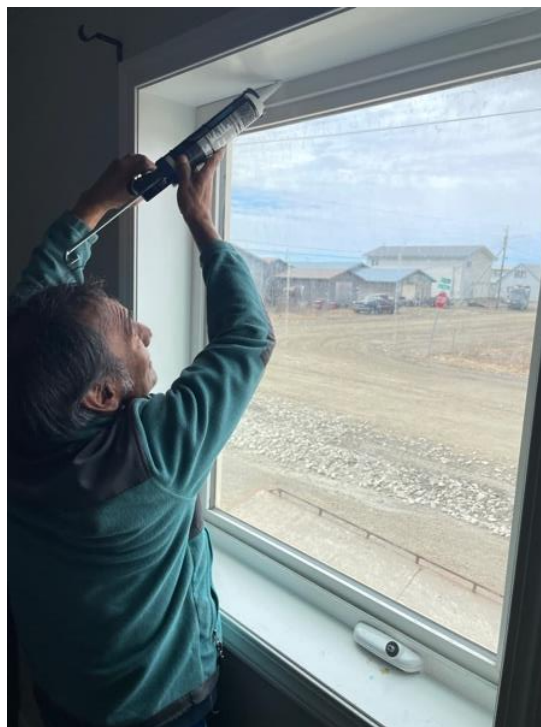
A workshop attendee learns how to weatherize an apartment in Nome, Alaska. Photo: Tyler Katzmar/REAP
