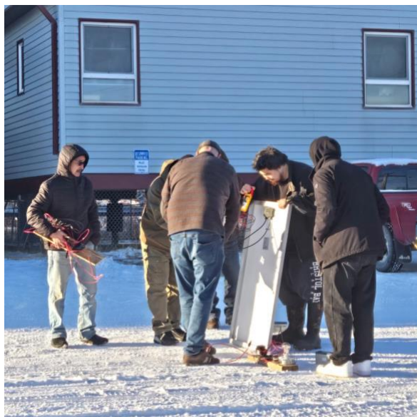
Instructors and students practice wiring a solar panel during a weeklong training in Bethel. Photo: Jacob Ivanoff
